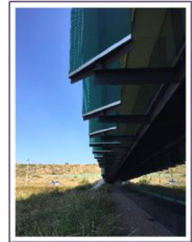
Member Photo: Desalination Plant © Hazel Zander iPhone 6, f/2.2, 1/942s, ISO-32, Equiv. 29mm
